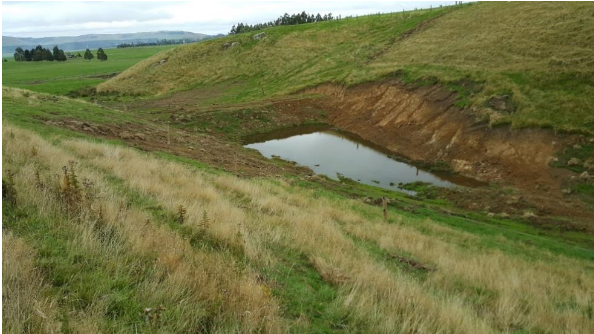
Figure 1: Typical example of a sediment trap with a bund, outlet to one side, keyed in to prevent leaks and located in a critical source area that will collect water from rainfall.
