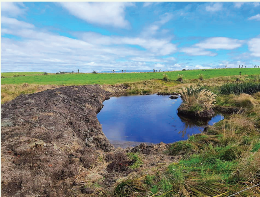
IMAGE 14: Bund at the bottom of the catchment immediately post construction looking east – January 2022.
