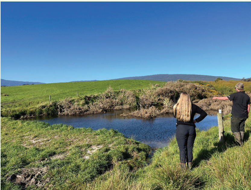
IMAGE 12: Bund located to the north of the dairy shed- Image taken during site visit in October 2022. Bank has been planted out in flaxes.
