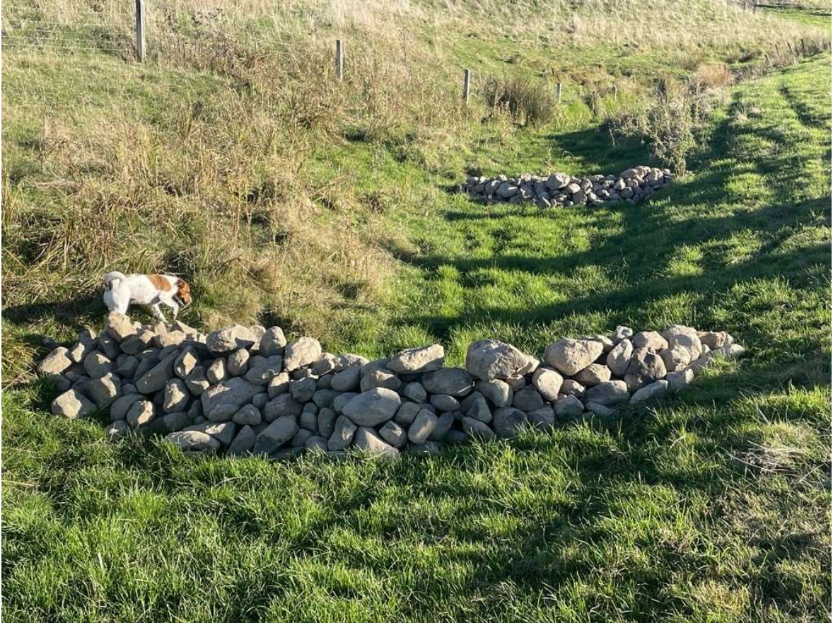
Figure 19. Illustration of check dams used to slow water into wetlands
