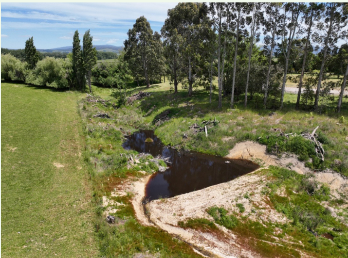
IMAGE 5: A bund has been placed to slow water flow allowing sediment to settle. The containment area for this series is shaped to aid in reducing water velocity. As with the other sites, the outlet is located to the side of the structure to ensure flow is disrupted and minimise the risk of blow out.
