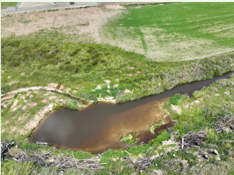
IMAGE 3: A close up of the first and larger sediment trap in this series of two. A bund has been placed to slow water flow allowing sediment to settle. Here you can see more definition of the depth of the sediment trap, and the overflow/outlet to the side of the containment area. The outlet is located to the side of the structure to ensure flow is disrupted and minimise the risk of blow out.
