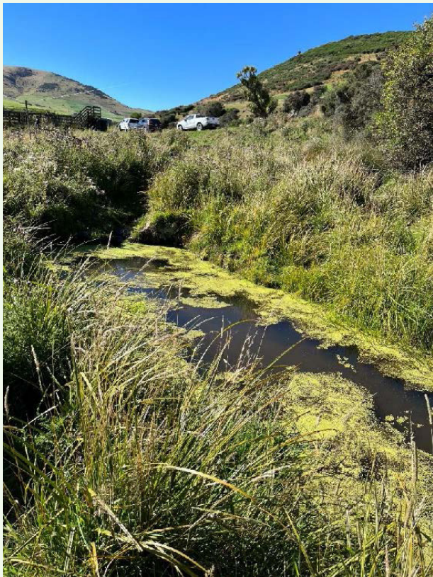
Image 2: The second sediment trap area in a series of two. Water movement through this sediment trap is slow. Discharge from the outflow flows over a heavily vegetated area before reaching an adjacent stream.
