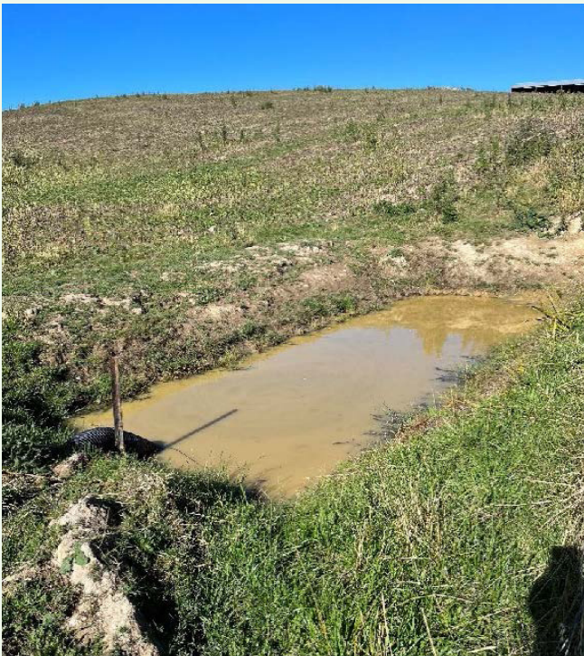
Image 3: The recently constructed sediment trap located next to a main access track. Track runoff flows into the top of the trap allowing the velocity to slow and sediment to drop out before flowing out via a tile drain. This image was taken after recent rain with evidence of finer sediments still suspended in the water.
