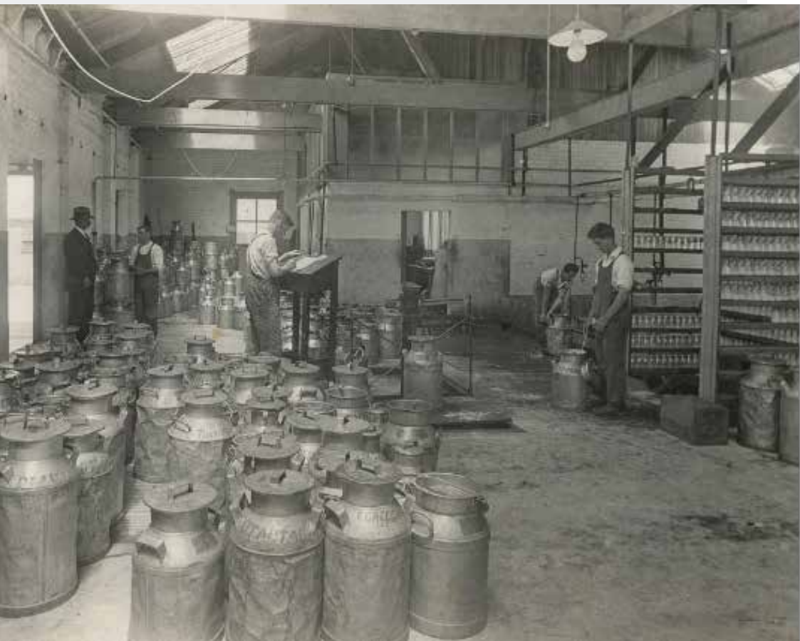
FIG 12. natlib.govt.nz | Men tipping cream, Edendale Dairy Factory
