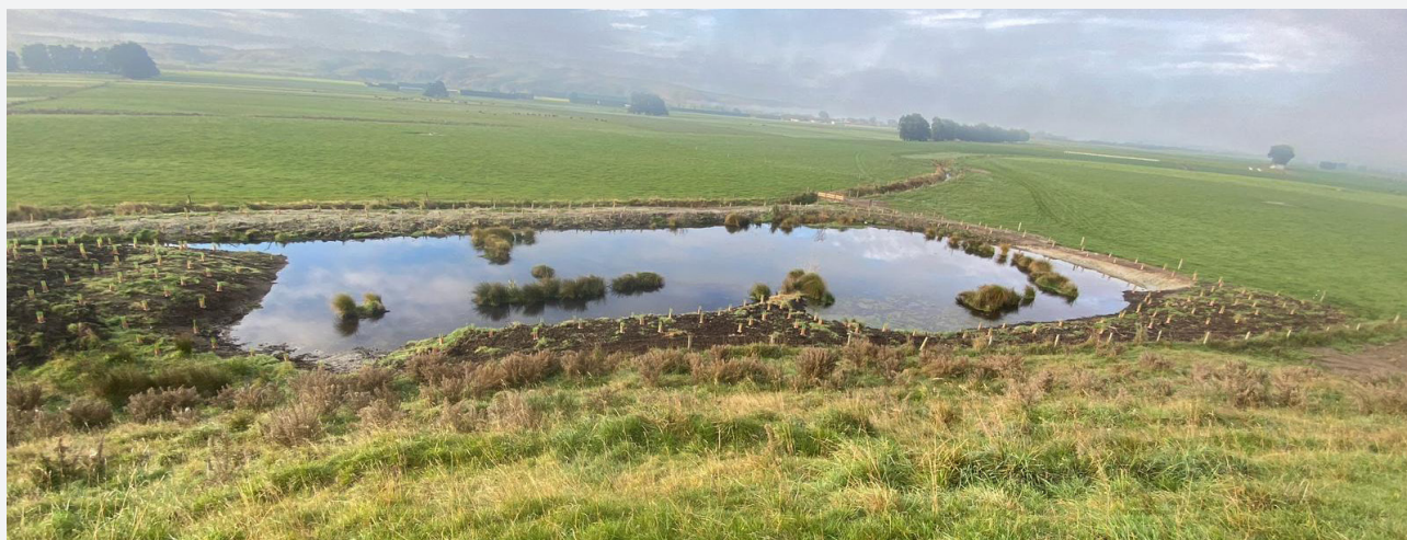
Enhanced existing duck pond converted into a treatment wetland.
