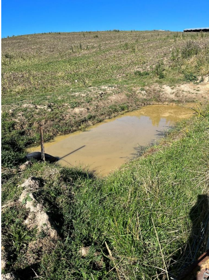
Image 3: The recently constructed sediment trap located next to a main access track. Track runoff flows into the top of the trap allowing the velocity to slow and sediment to drop out before flowing out via a tile drain. This image was taken after recent rain with evidence of finer sediments still suspended in the water.
