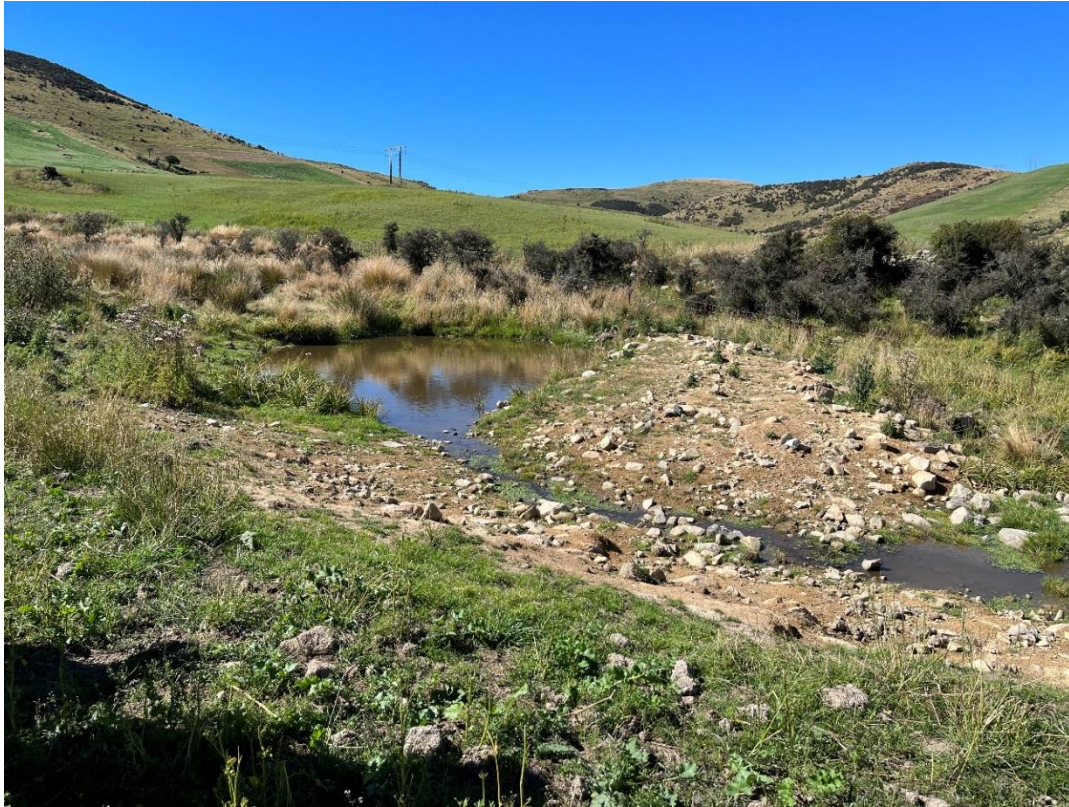
Image 1: A bund has been placed to slow water flow allowing sediment to settle. The outlet is located to the side of the structure to ensure flow is disrupted and minimise the risk of blow out.
