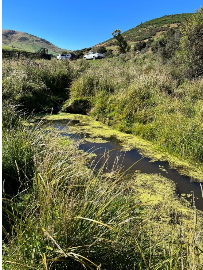
Image 2: The second sediment trap area in a series of two. Water movement through this sediment trap is slow. Discharge from the outflow flows over a heavily vegetated area before reaching an adjacent stream.
