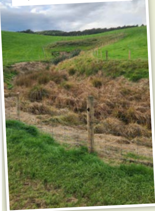
During: new fence partially erected
